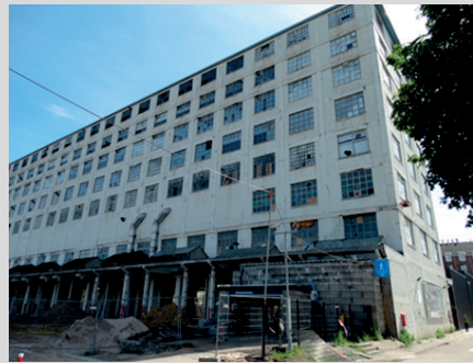
Sphinx building: former industrial building, currently under renovation for student hotel
