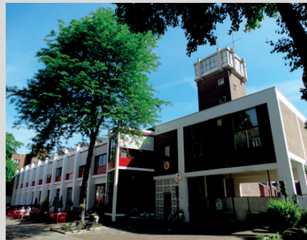
De Brandweer: former fire station, now it is a multifunctional building for start-ups, offices, a restaurant and meeting place for social events
